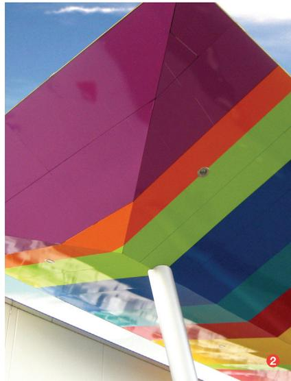
Using Avery® 900 Supercast film, the installation was completed very quickly, proving once again that vinyl is quicker to apply than paint.
